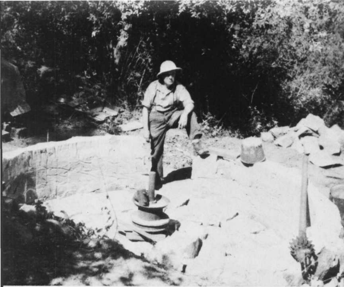
The author's father at his partially completed arrastre, built in 1948 at Big Oak Flat, California. Indians were using arrastres when Spanish arrived.
